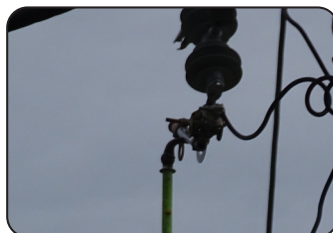
A lineman putting the fuse back in place with a hot stick. Close up below.
