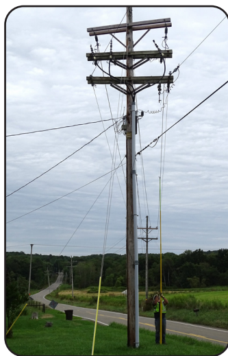
A lineman putting the fuse back in place with a hot stick. Close up below.
