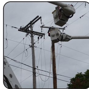
Equipment transferred from the old pole to the new pole.
