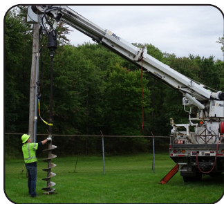
Setting an anchor for a guy wire with the digger truck.
